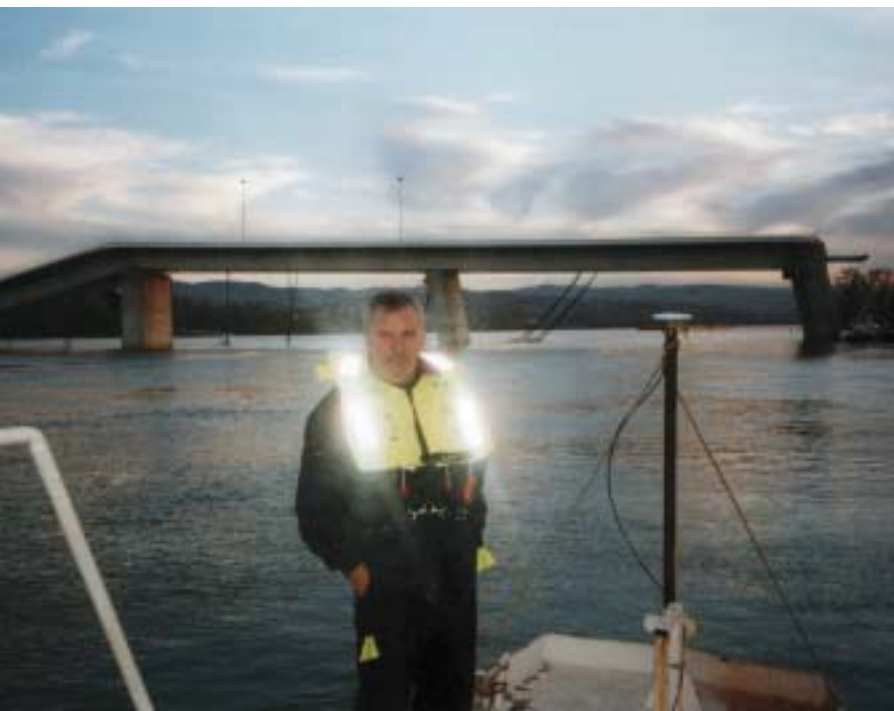
Professor Ninkov stands before a damaged bridge during hydrographic measurements.
