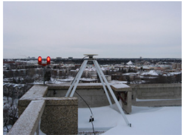
Stantec network reference station located on the roof of the Stantec head office in Edmonton. The station consists of a Trimble Zephyr Geodetic™ antenna (shown) connected to a Trimble NetRS receiver.
